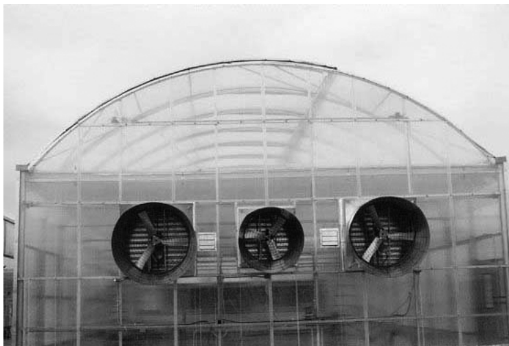
Figure 12.12 Large ventilation fans placed at the end of the greenhouse. The size and number of exhaust fans will determine the amount of air that will be exhausted from the greenhouse. In this situation, this greenhouse was located in a warm climatic region; therefore, a need for high capacity air movement existed.
