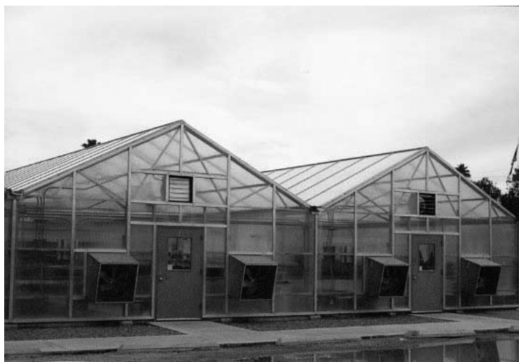
Figure 12.2 Gutter-connected multiple-bay greenhouse. The number of bays can be many depending on the designed use, with each bay gutter-connected.
