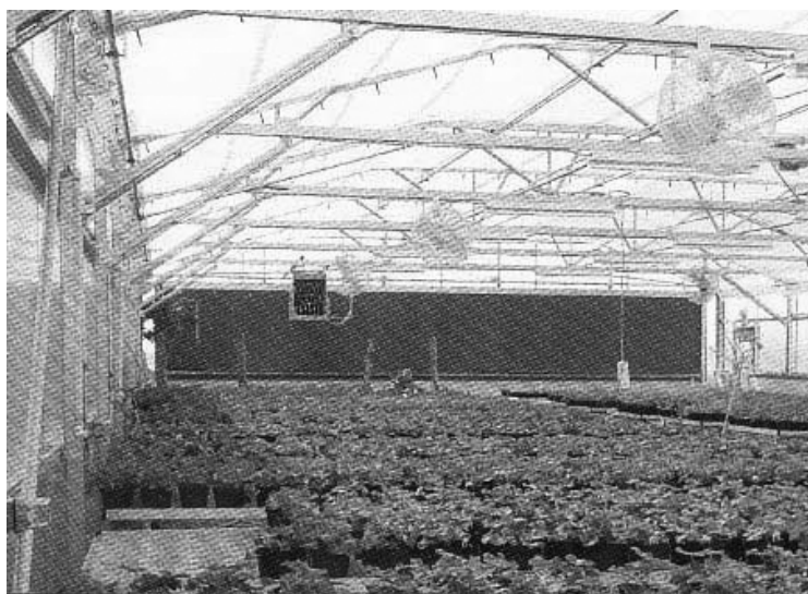
Figure 12.13 The cooling pad in this greenhouse occupies the entire end of the greenhouse. The size of the cooling pad can significantly affect the cooling effect.
